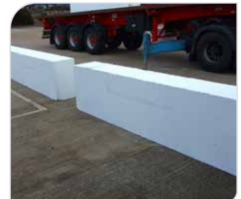
Offloading of 4m concrete barriers
