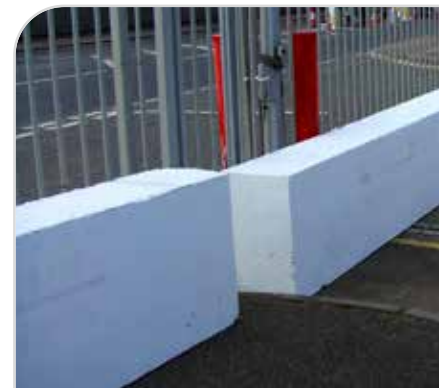
4m concrete barriers blocking entrance
